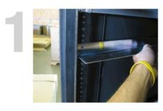
Install the support rail between the rack rails from inside the rack. The supplied screw will only fit in every third hole which corresponds to a rack space.
