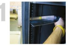
Install the support rail between the rack rails from inside the rack. The supplied screw will only fit in every third hole which corresponds to a rack space.
